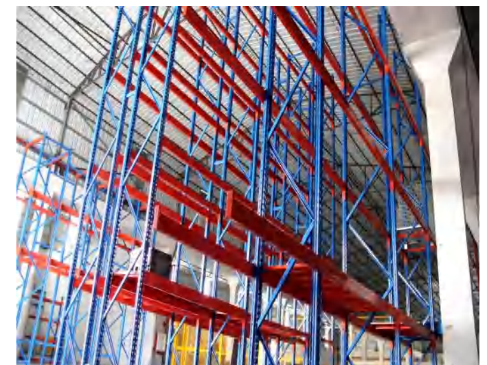
Drive-in rack project 驶入式货架案例
