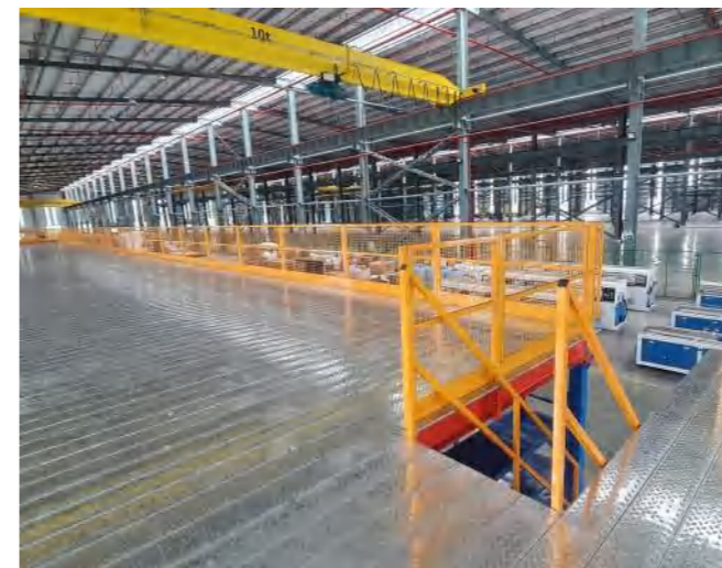
Mezzanine floor with steel gusset plate 钢平台铺钢扣板
