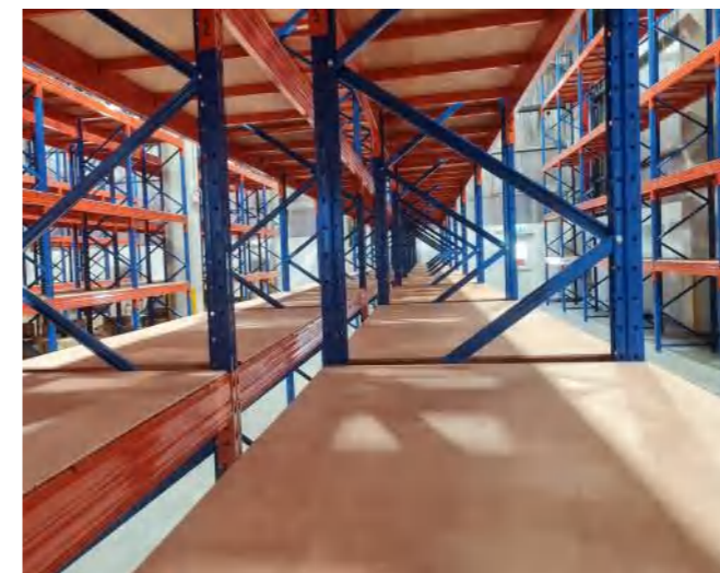
Rack with plywood 货架铺木板
