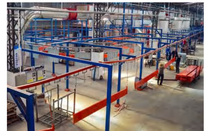
Painting line 喷涂线
