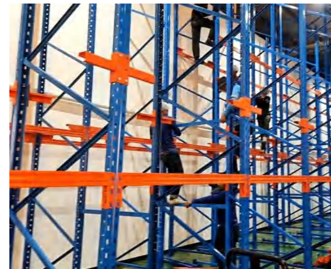
Drive-in rack project 驶入式货架案例
