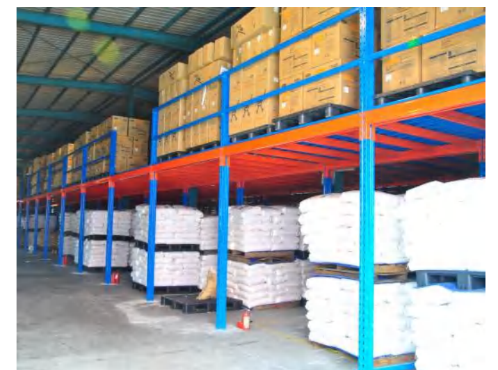
Mezzanine floor project 钢平台案例
