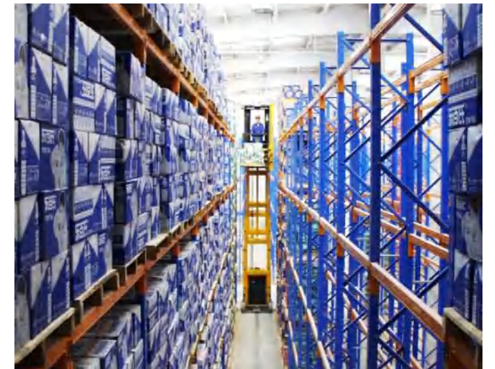
VNA rack project 窄巷式货架案例
